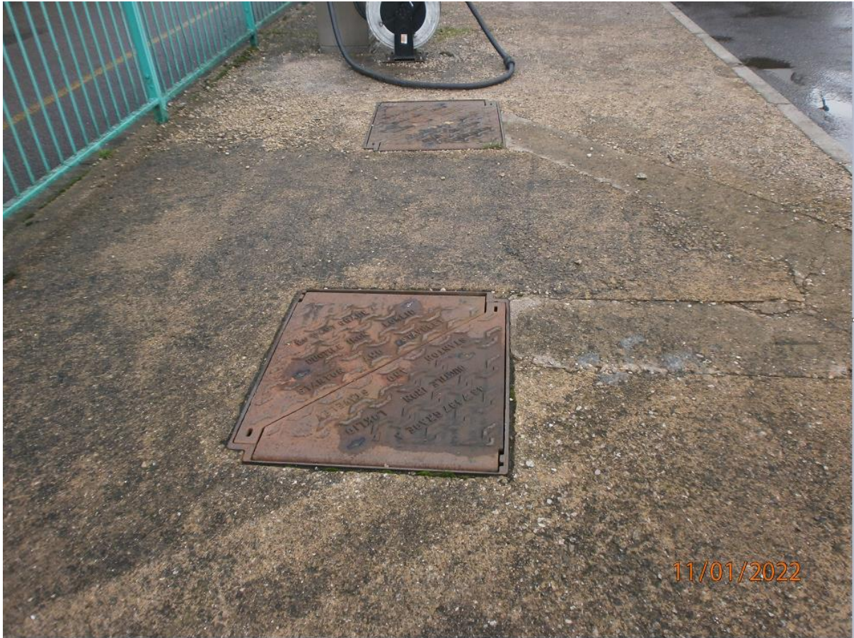
Photograph of Gas Oil Storage
